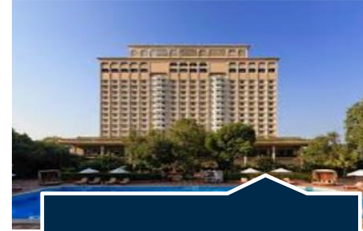
The Taj Mahal, New Delhi No supply in Heart of Central Delhi
